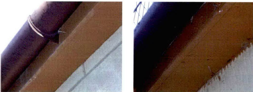
Figs. 13 & 14 Boxed soffits tightly fitting against the rear wall
