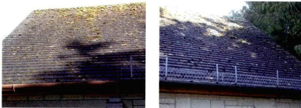
Figs. 7 & 8 Roof and ridge tiles to the rear
